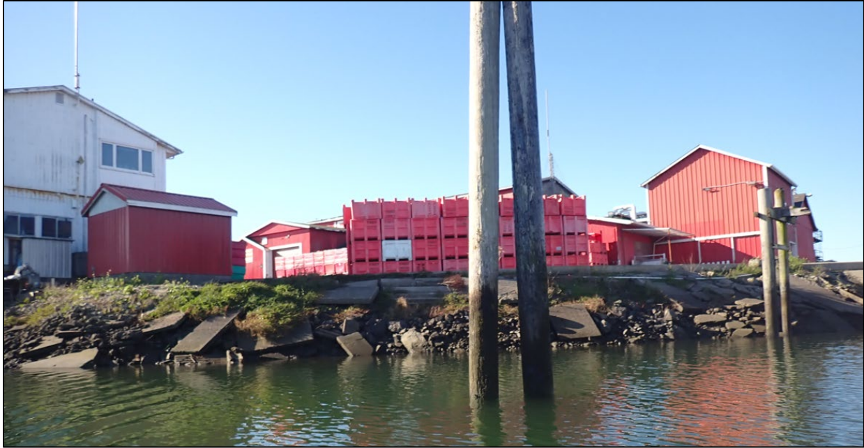
Figure 5. Riprap Shoreline to the South of the Bulkhead Wall
