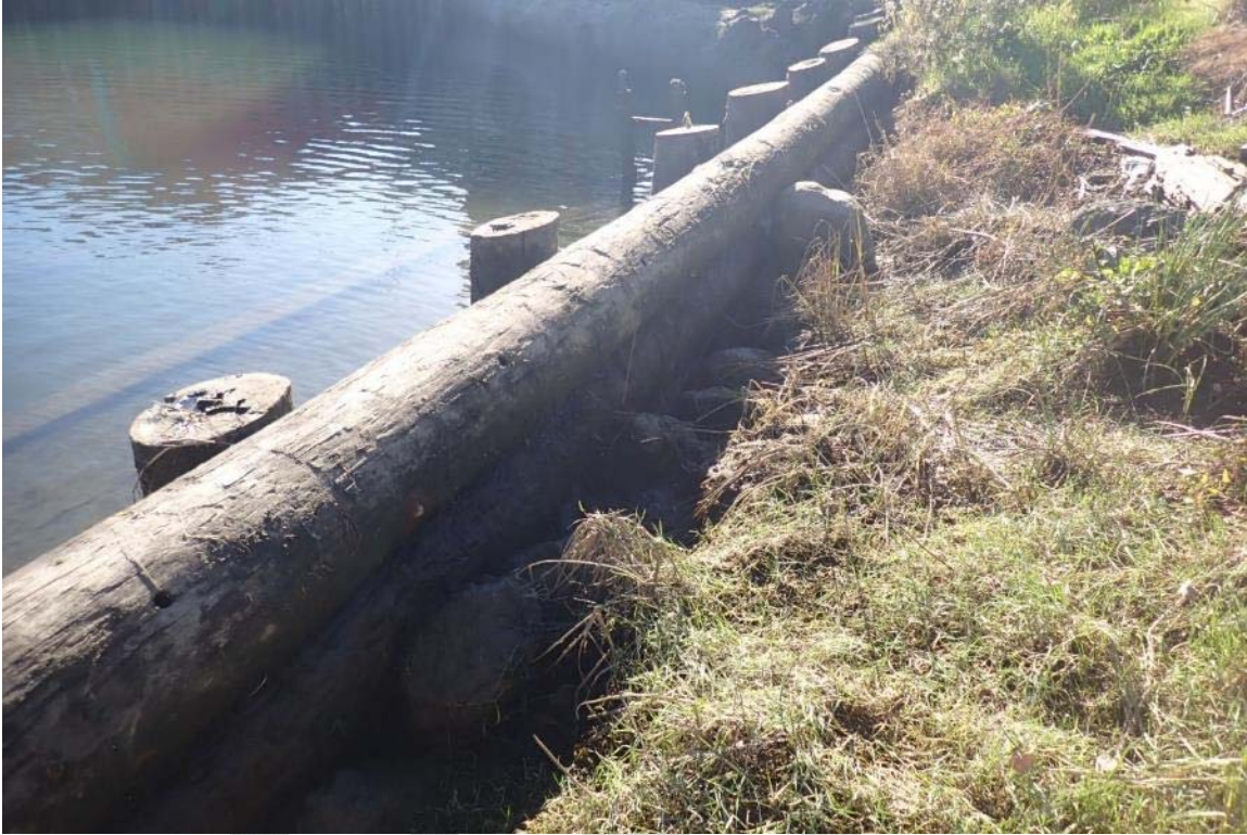
Photograph 22: North Bulkhead Lagging
