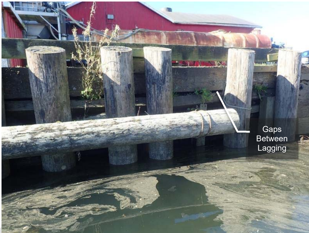
Photograph 19: East Bulkhead Lagging
