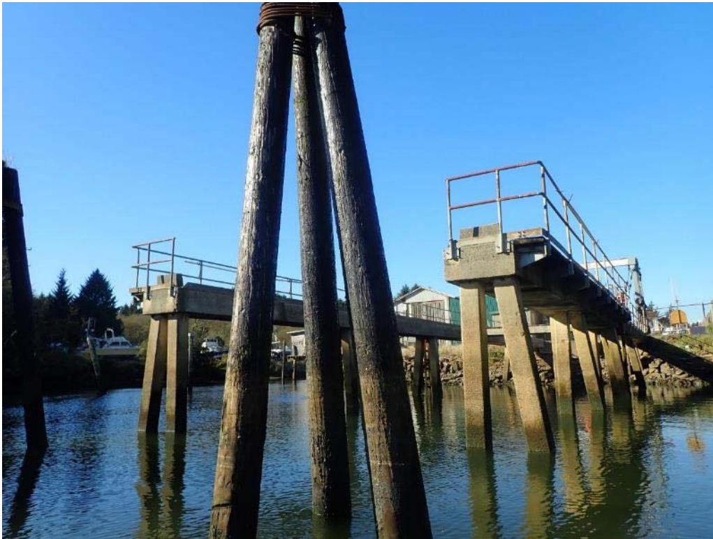
Photograph 12: Typical Timber Pile Dolphin
