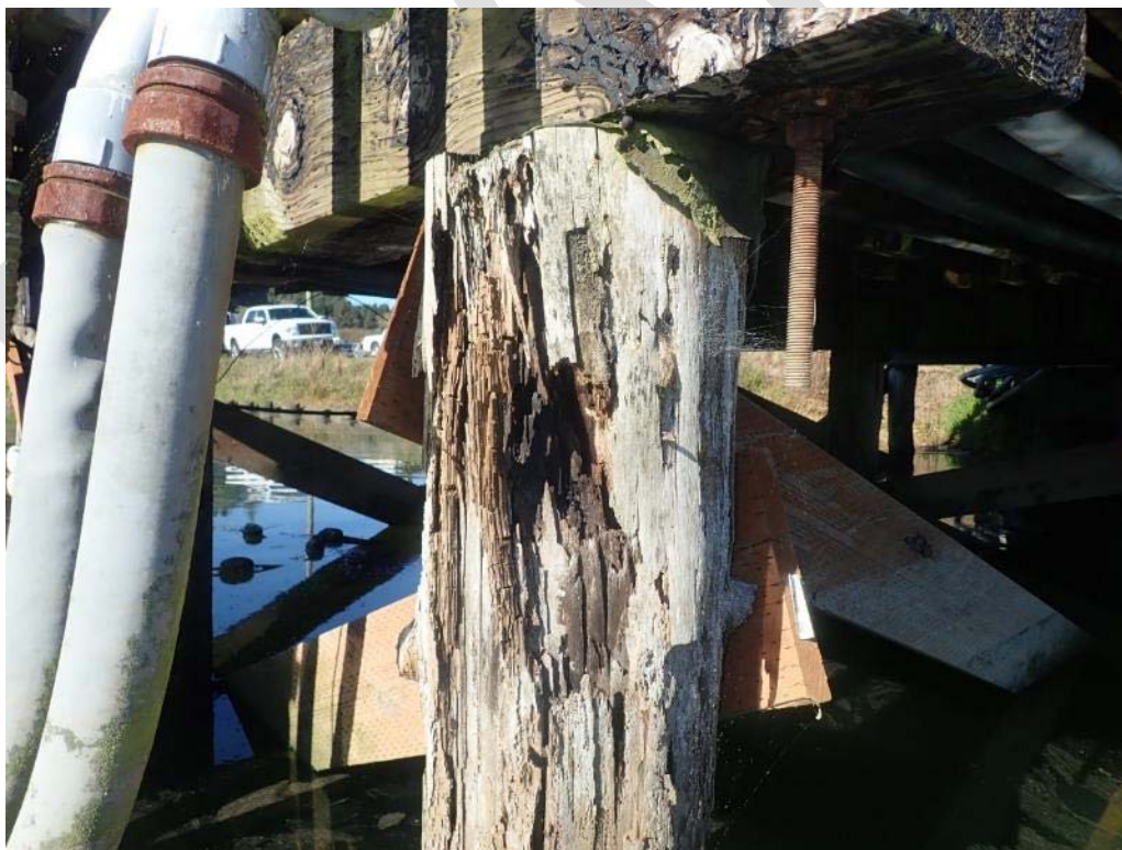
Photograph 29: West Access Pier Timber Pile 4:C with Severe Section Loss
