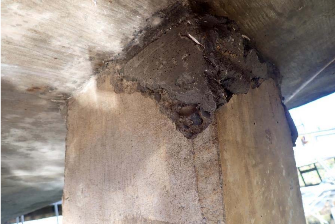
Photograph 5: Corner Spall Repair on Pile 2:A
