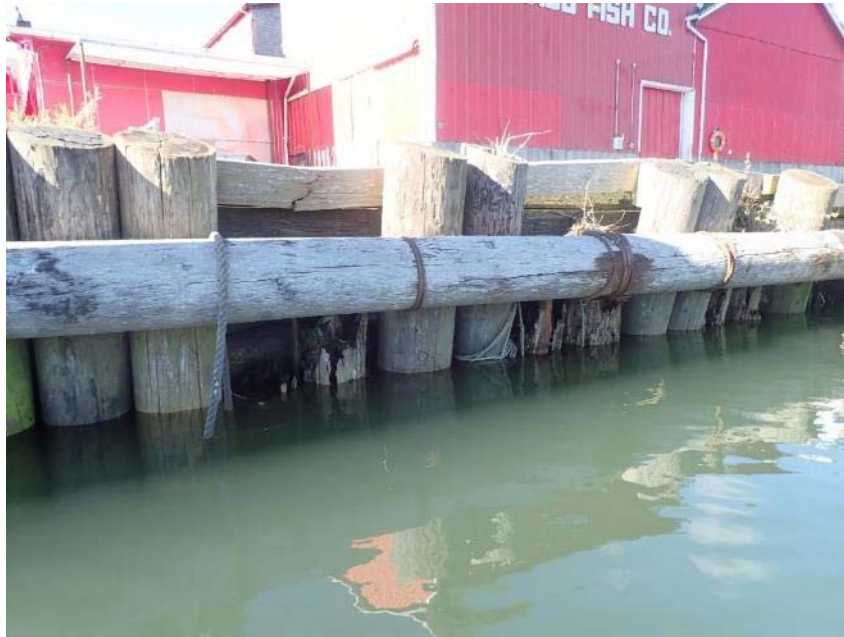
Photograph 17: East Bulkhead Piles
