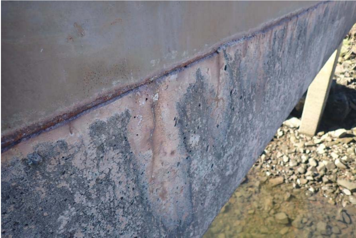
Photograph 8: Typical Cracking Beneath Wheel Guide/Kick Plate
