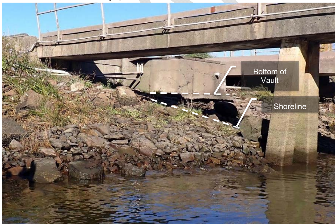
Photograph 15: Erosion Evident Below Concrete Vault
