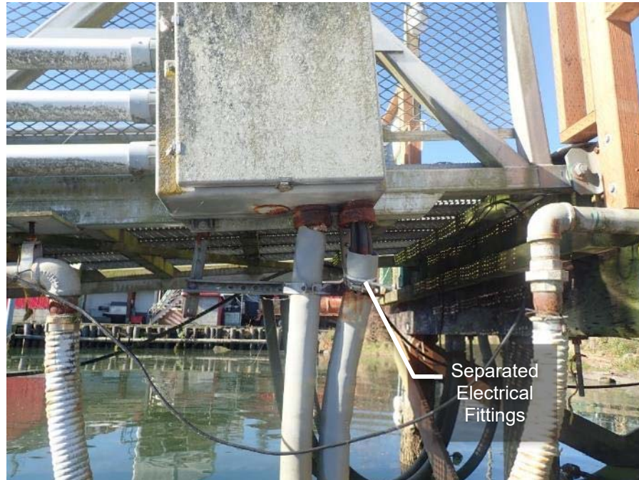
Photograph 36: West Access Pier Electrical Utilities
