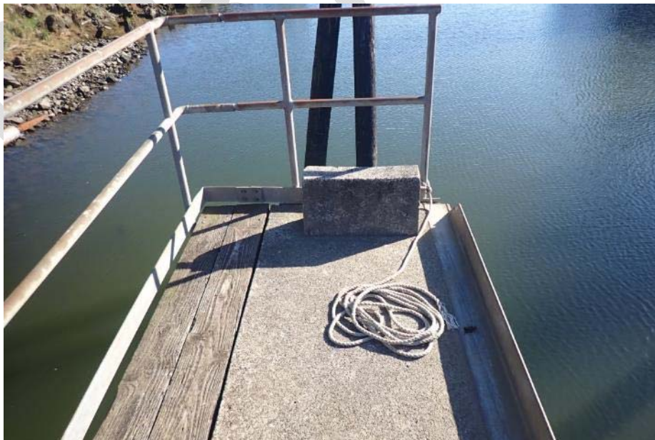
Photograph 10: Typical Handrail with Minor Corrosion
