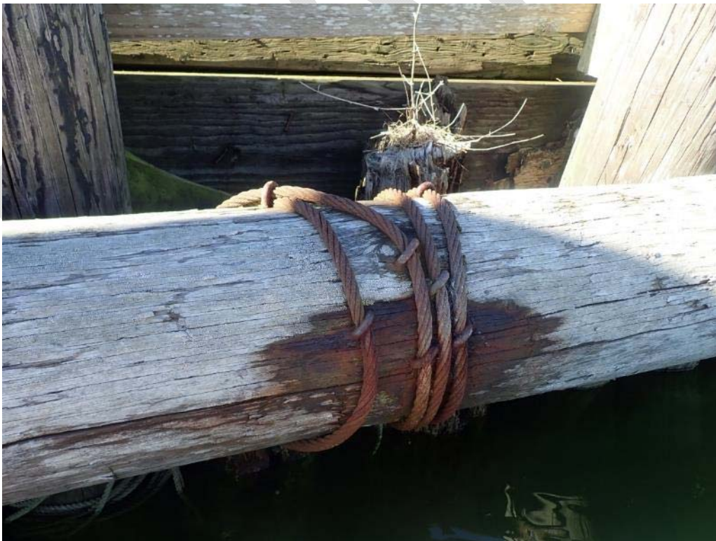
Photograph 21: East Bulkhead Tieback Strands
