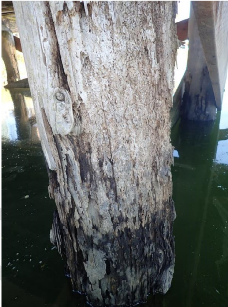
Photograph 27: West Access Pier Typical Timber Pile with Shell Delamination
