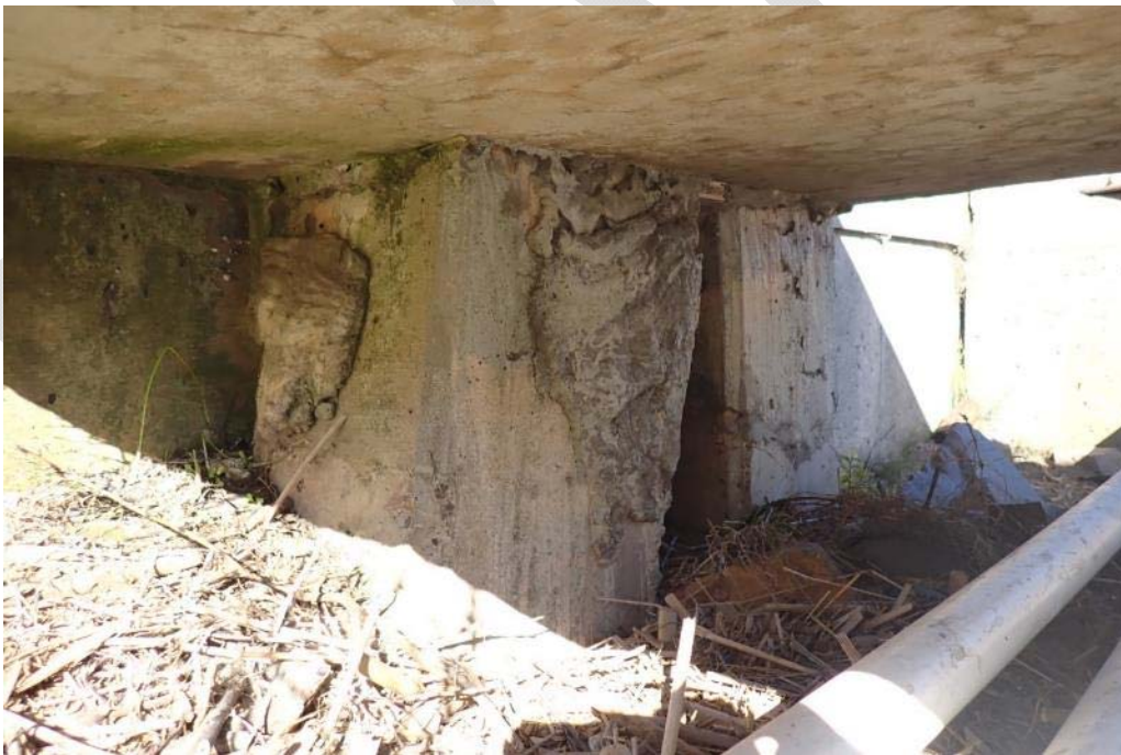
Photograph 4: Corner Spall Repair on Pile 1:A
