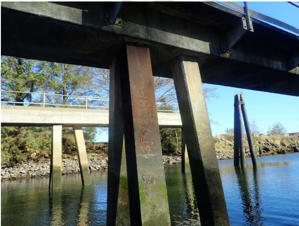
Photograph 6: Steel H-Pile at Bent 5:A
