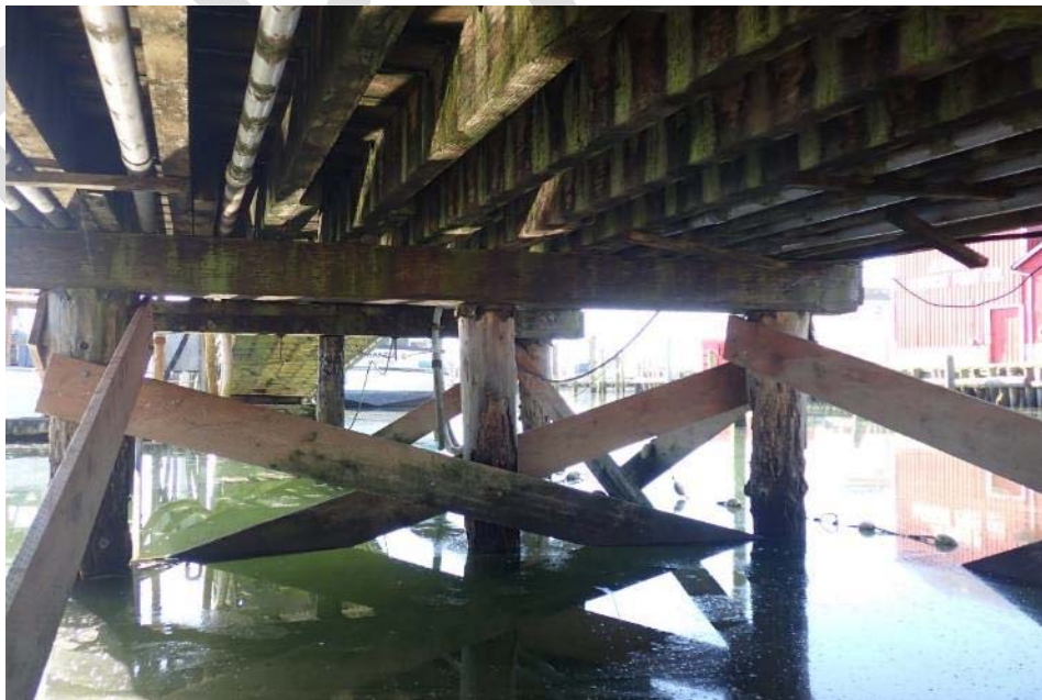
Photograph 33: West Access Pier Timber Cross Bracing
