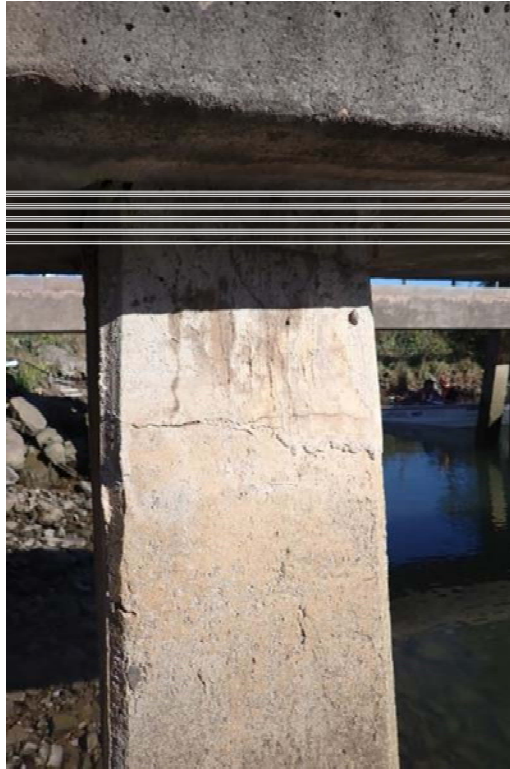
Photograph 3: Moderate Cracking on Pile 2:A
