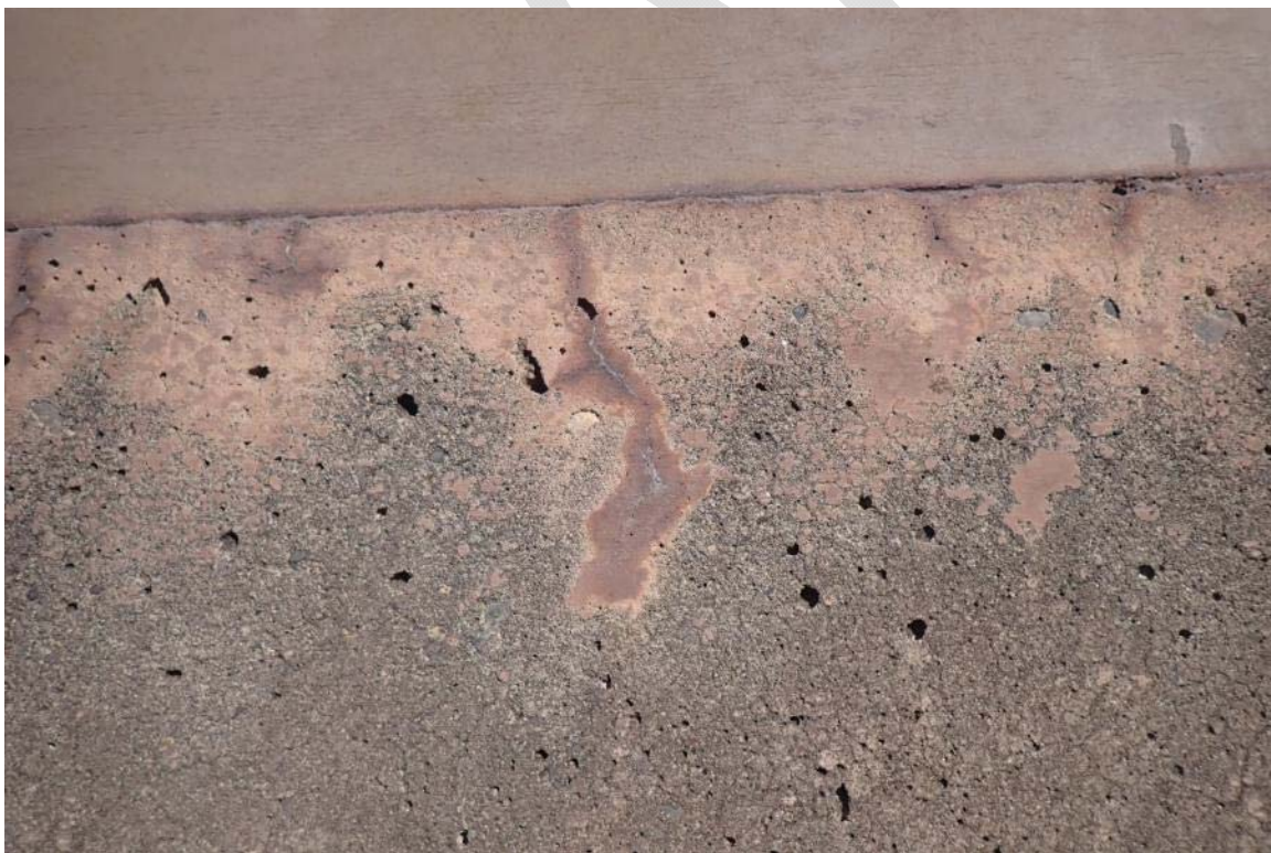
Photograph 9: Typical Cracking and Rust Staining
