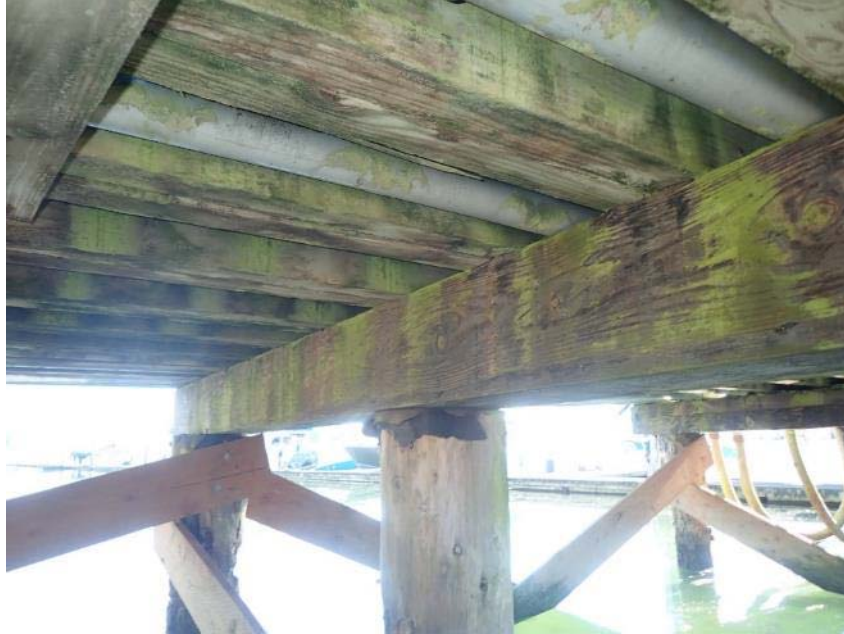
Photograph 32: West Access Pier Timber Stringers
